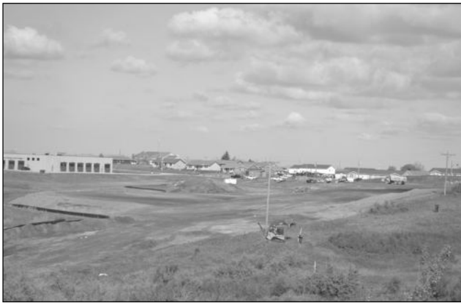
Construction started on new community center.
