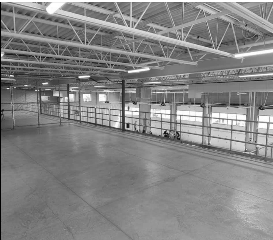
Here is another spacious room it is on the top level. We aren't sure as of this day what this space will be used for. I am sure the EMS and Fire Dept will have some good use for this space. The whole building was awesome.
