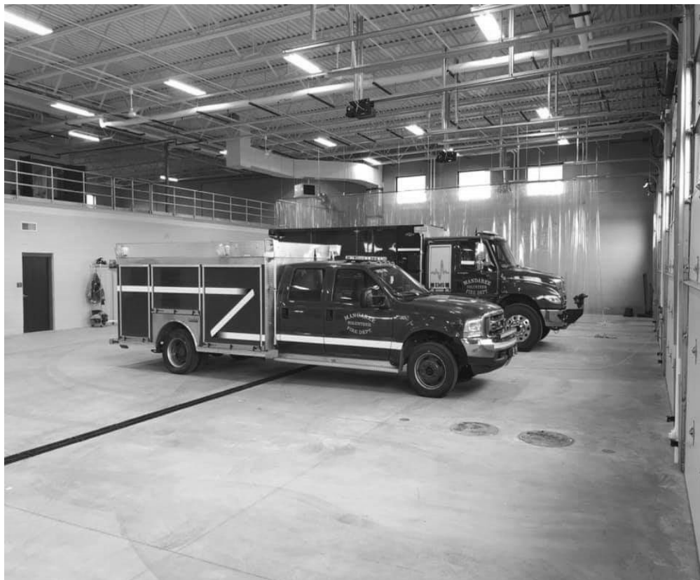
On the other side of the facility the Mandaree Volunteers Fire Trucks are parked inside the same building as the ambulances. As you can see the spacious room they have for their emergency vehicles.
