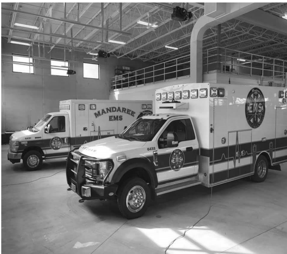
The EMS Ambulance crew now has a home for their ambulances which are pictured above. The building is very clean and refreshing to know these ambulances will be in good care from the elements.
